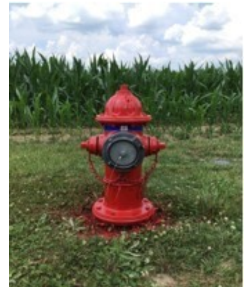
Repainted and NFPA Color Coded Fire Hydrant
