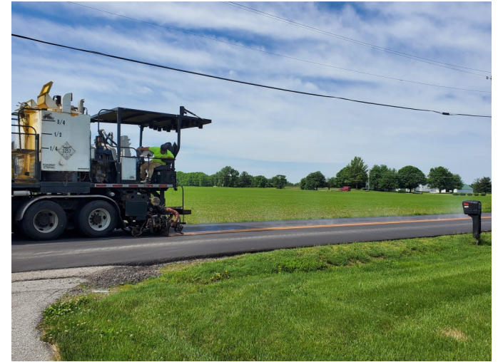
Whitestown Parkway Striping after Resurfacing
