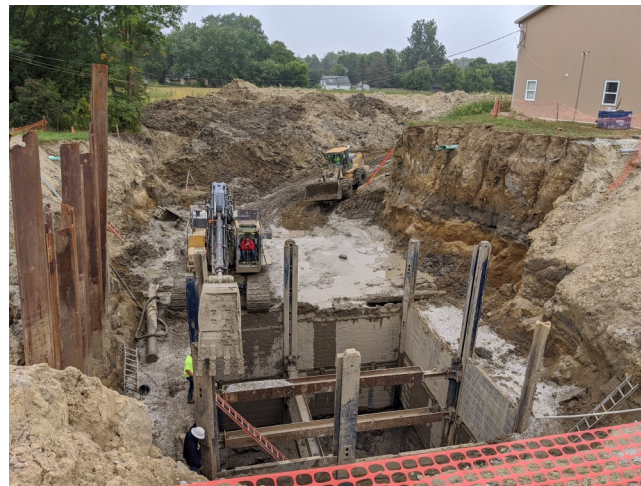
Whitestown Lift Station During Construction
