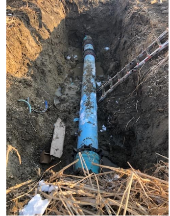
16" Water Main Break Repair
