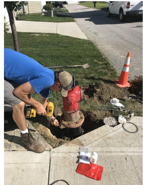
Raising Fire Hydrant
