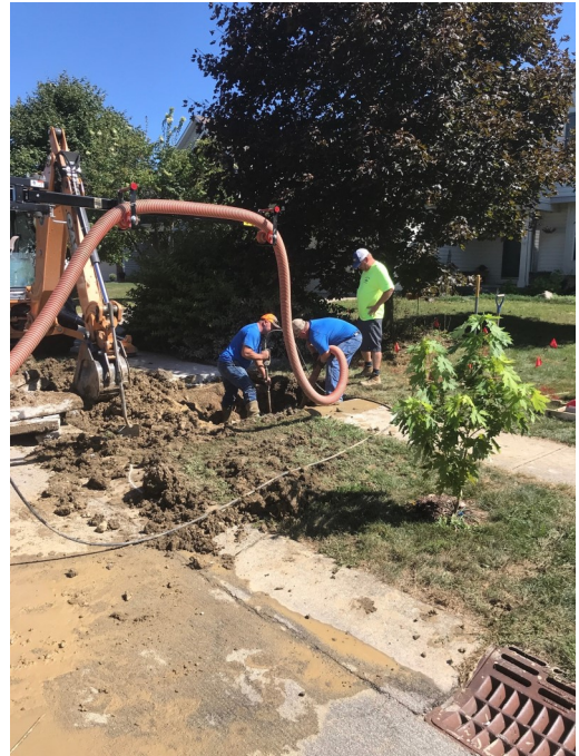
Replacing Service Line
