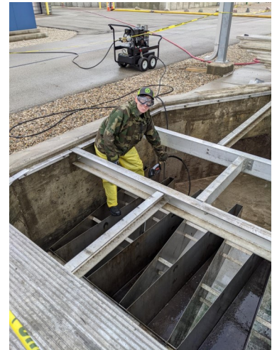
Tank Cleaning at WWTP
