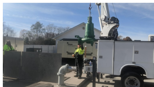
Royal Run Lift Station Pump Installation
