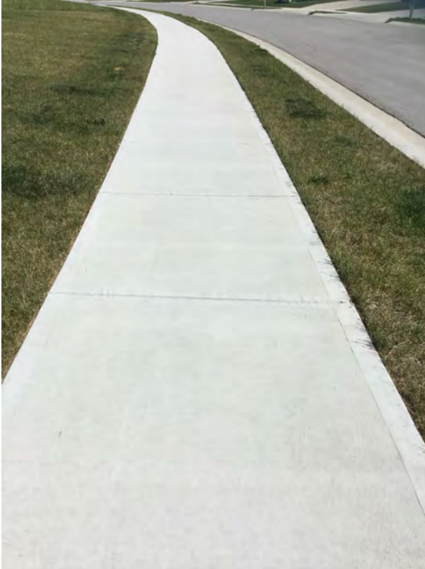
Source: HWC Engineering
