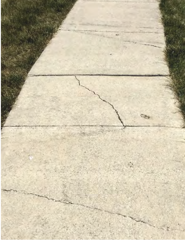
Source: HWC Engineering
