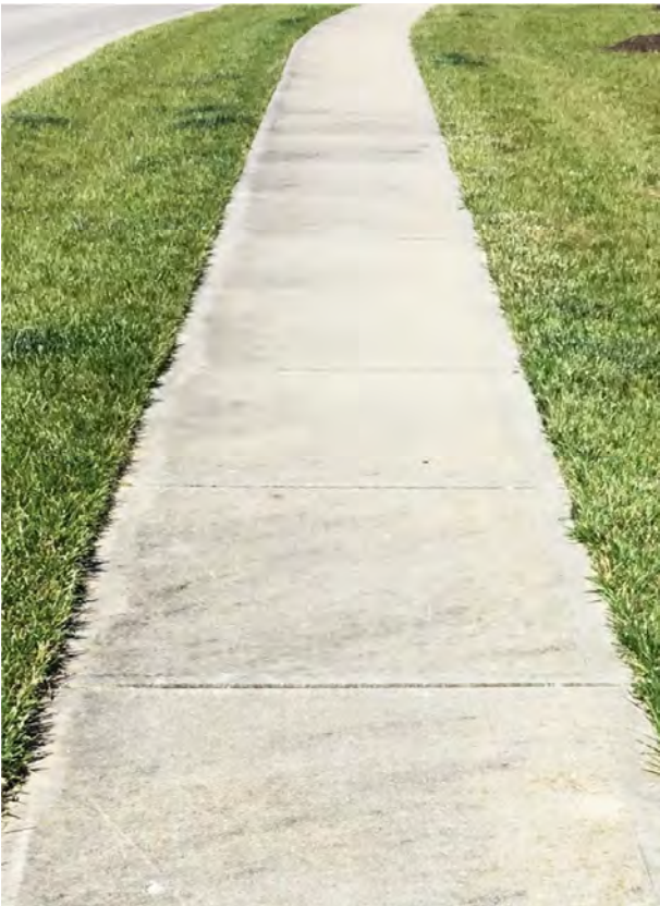
Source: HWC Engineering
