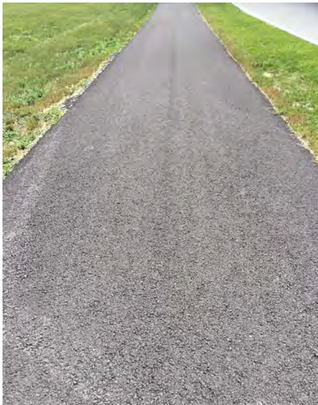
Source: HWC Engineering
