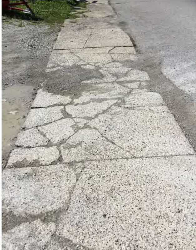
Source: HWC Engineering
