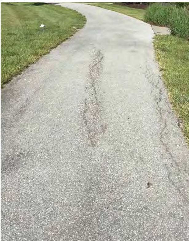
Source: HWC Engineering
