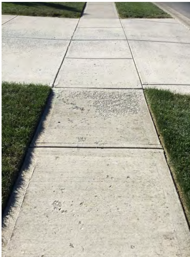
Source: HWC Engineering
