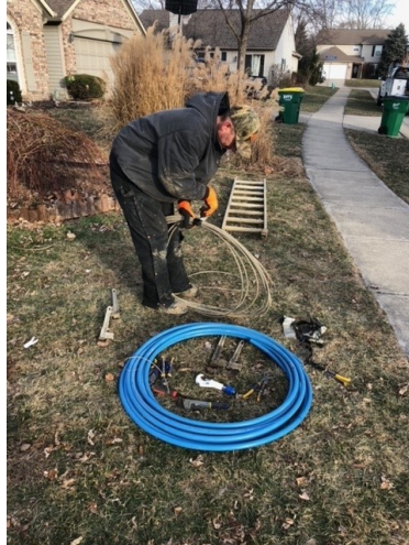
Prepping for Water Service Line Repair
