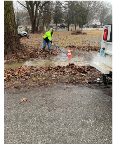
Cleaning Clogged Storm Drain
