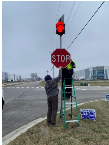
Installing flasher On Stop Sign at Albert S White and CR 500 E
