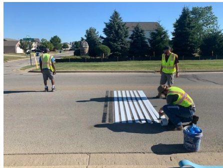
Rumble Strip Installation
