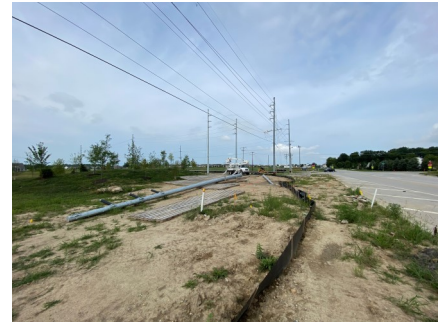
Beginning of Utility Relocation for Main Street RAB
