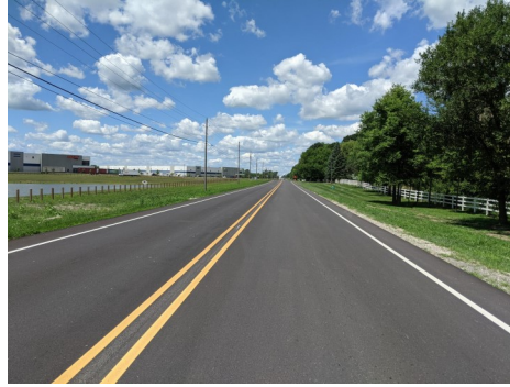
Indianapolis Rd Resurfacing for Community Crossings Grant
