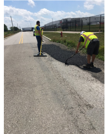
Repairing Potholes
