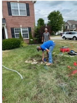
Water Meter Replacement
