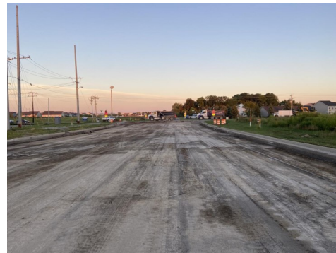
Albert S White Dr and Main St Roundabout Construction
