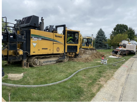
Boring Forcemain for Main Street Lift Station
