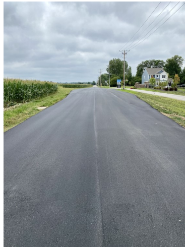
Paving on CR 700 E
