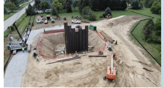
Main Street Lift Station Construction
