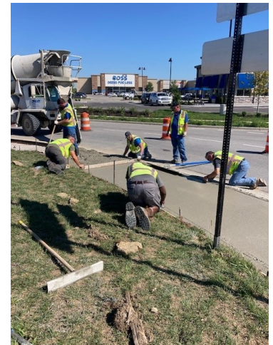
Installing Truck Apron on Mills Roundabout
