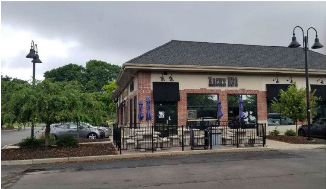
(Illustrating masonry detail and building materials comprising the body and sloped roof)
