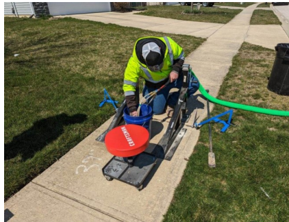
Repairing a Sunk Sidewalk Using the Sidewalk Jack.
