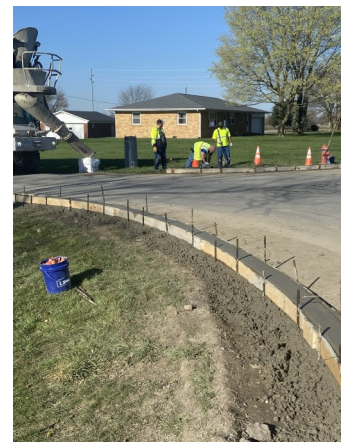
Curbs Placed on CR 575 E and Pierce St
