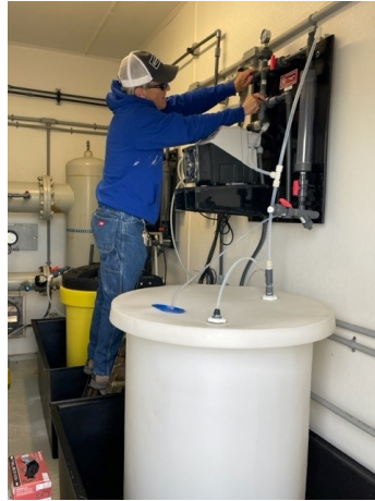
Booster Pump Station Preventative Maintenance
