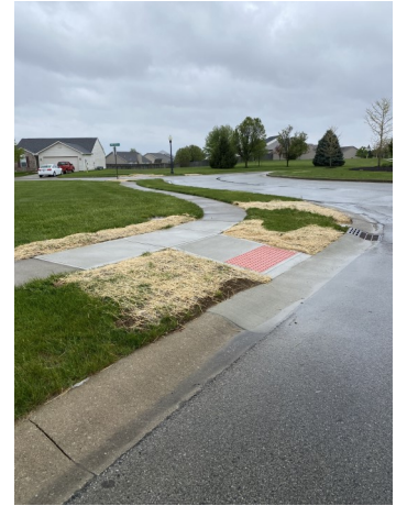
ADA Compliant Curb Ramps in Walker Farms
