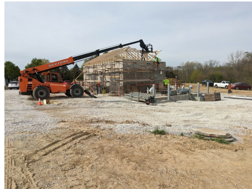
Main Street Lift Station Construction
