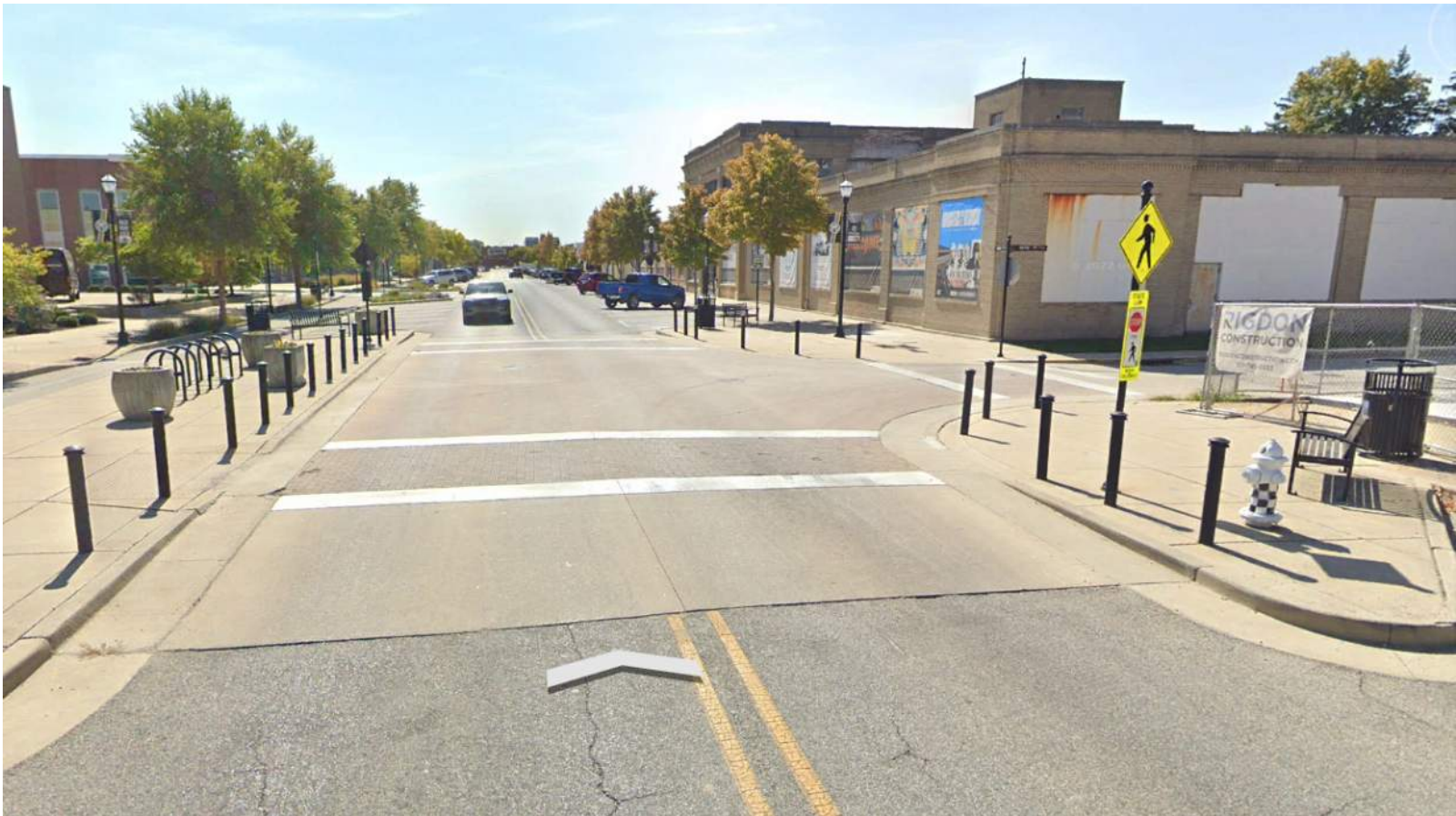
Main Street - Speedway, IN Raised Intersection
