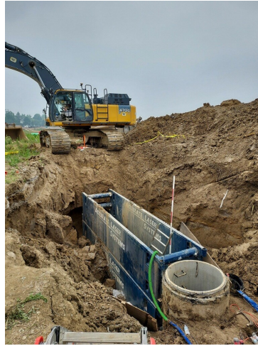
Connecting manholes for Jackson run
