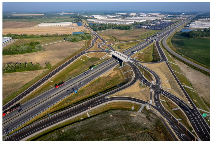
Midpoint Interchange over I-65 at exit 131
