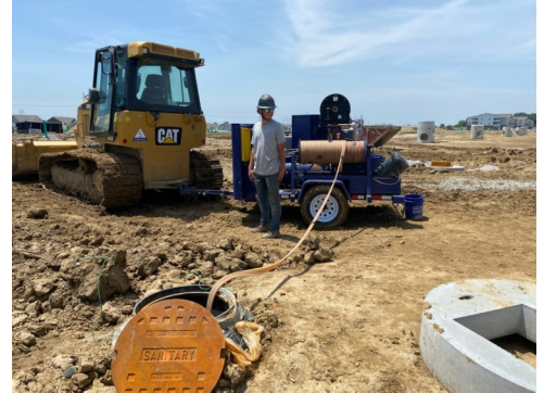
Testing manholes at Cottages of Bridle Oaks
