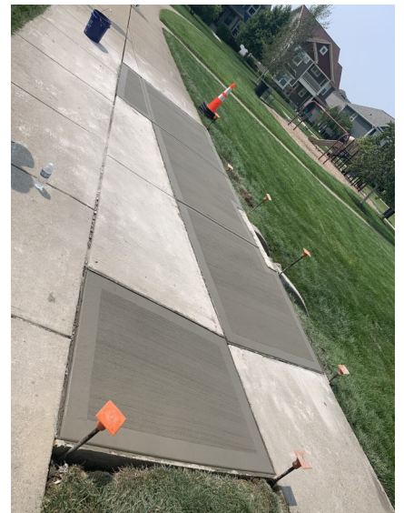
Repaired sidewalks in Clark Meadows
