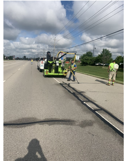
Crack Sealing on Whitestown Parkway
