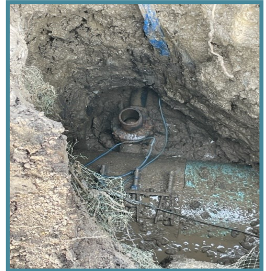
VALVE BOX REPAIR
