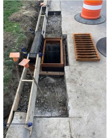
REPAIRING CURBS ON ANSON BLVD
