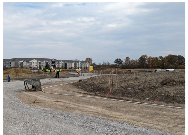
PERRY WORTH ROAD CONSTRUCTION
