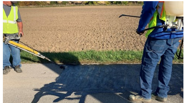
STREET DEPARTMENT CRACK SEALING CR S 450 E
