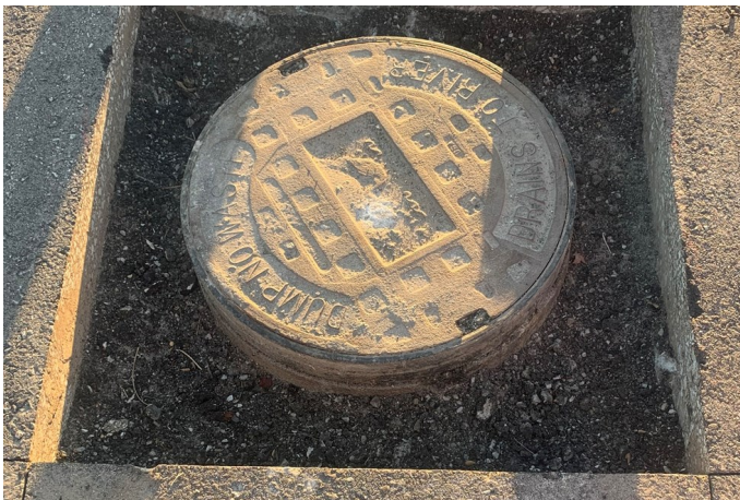
40 MANHOLE REPAIRS ON 450 S, 500 E, ANSON
