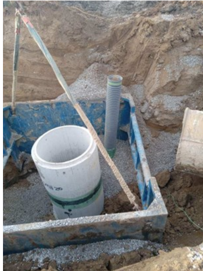
NEW SANITARY SEWER MANHOLE BEING INSTALLED IN BRIDLE OAKS
