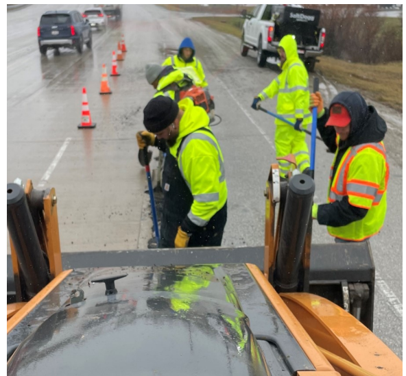
Filling Potholes on Whitestown Parkway
