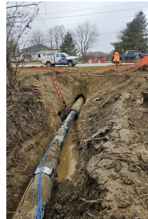
12" water main bore under 267
