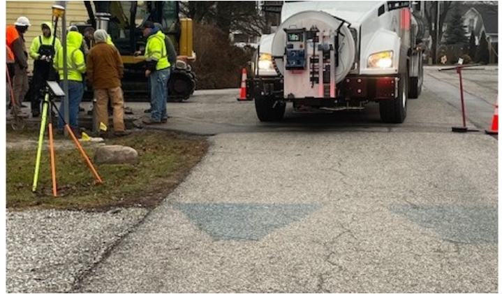
Water Main Break Repair at Neese and Bowers St
