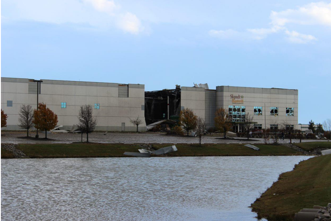
Figure 42. Image of tornado damage to Skjodt-Barret building in Lebanon, November 2013
