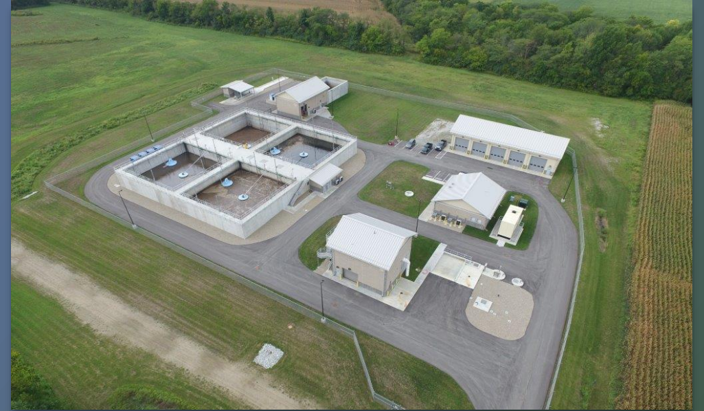
Whitestown Wastewater Treatment Plant
