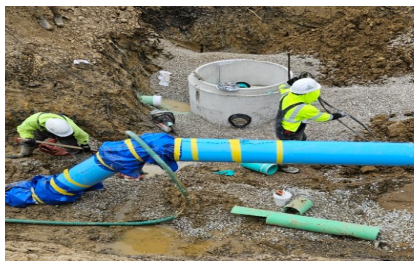
WATER MAIN BEING RAISED FOR A STORM CROSSING AT GREENVIEW APARTMENTS
