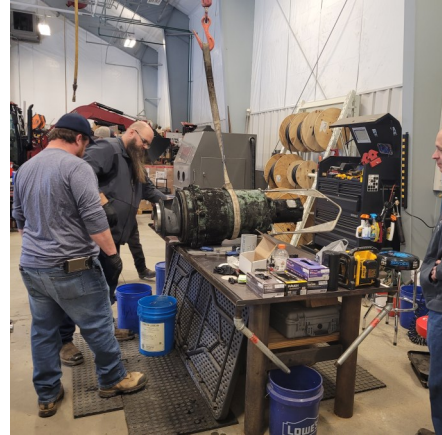
WASTEWATER REPAIRING A LIFT STATION PUMP
