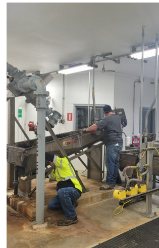
WASTEWATER REPAIRING THE GRIT CLASSIFIER
