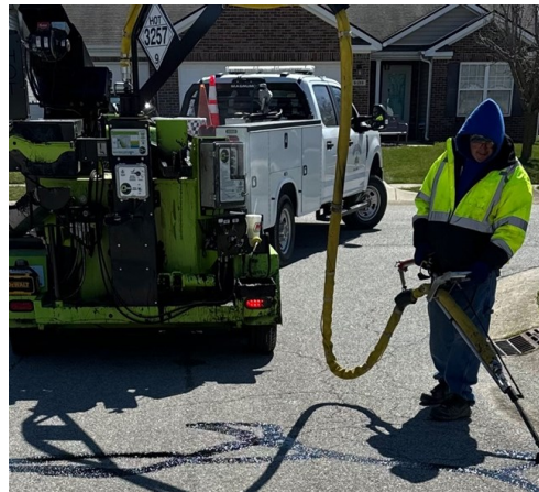
STREET DEPARTMENT CRACK SEALING IN WALKER FARMS
