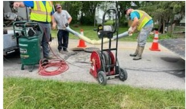
LINING SEWER MAIN THAT WAS DAMAGED ON PIERCE
