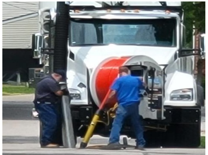
CLEANING SANITARY SEWER ON BOWERS ST
