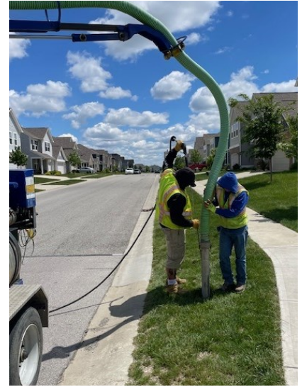
VACUUMING OUT HOLES FOR SIGNS
