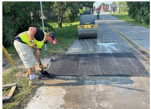
ASPHALT PATCH ON MAIN STREET FOR WATER MAIN
