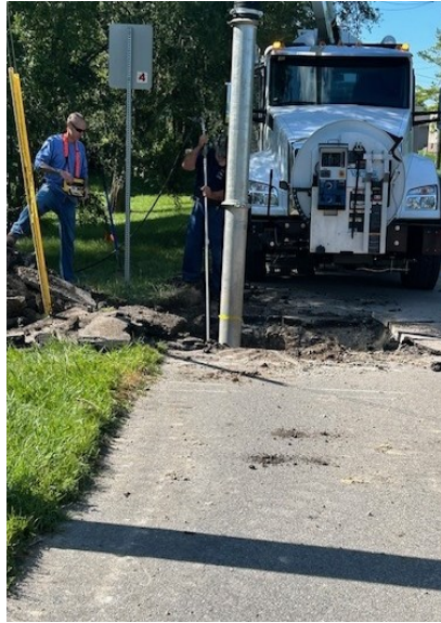
POTHOLING WATER LINE ON N. MAIN ST
