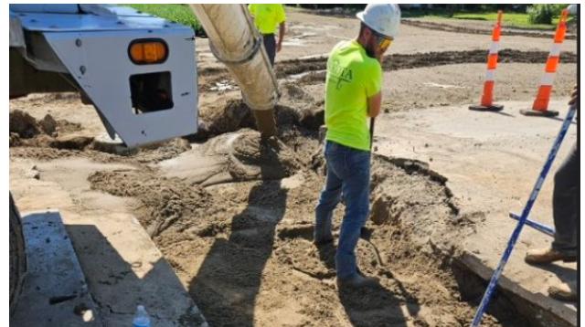
STORM CROSSING ON CR 450 FOR GREEN CYCLE
