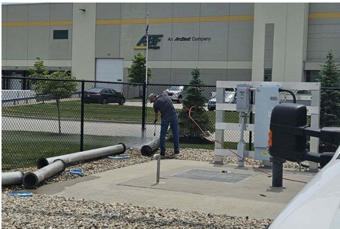
REPLACING VAC TUNES AT BUSINESS PARK LIFT STATION
