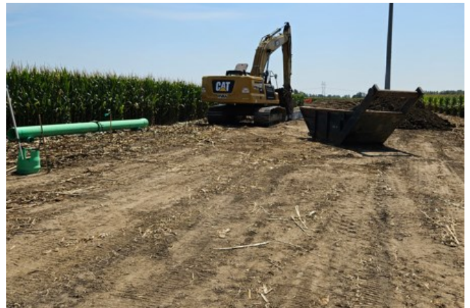
INSTALLING FORCE MAIN FOR PEABODY WEST
