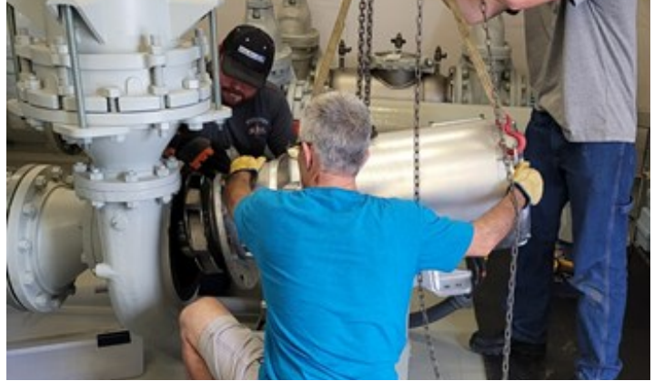
Installing Motor at Indy Rd Booster Station
