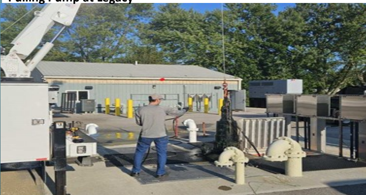
Pulling Pump at Legacy
