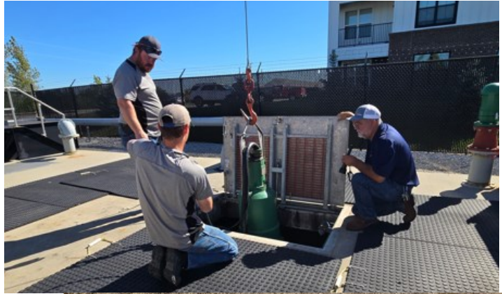
Installing Pump into Indy Road Pump Station
