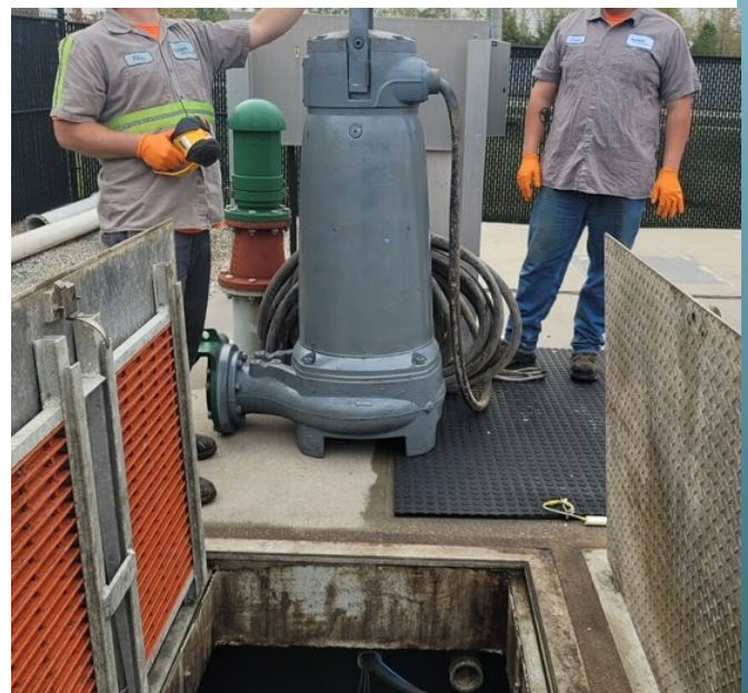
INSTALLING TEMP PUMP AT INDY RD LIFT STATION
