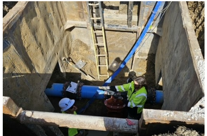
CUTTING IN A TEE FOR ILPNW BUILDINGS
