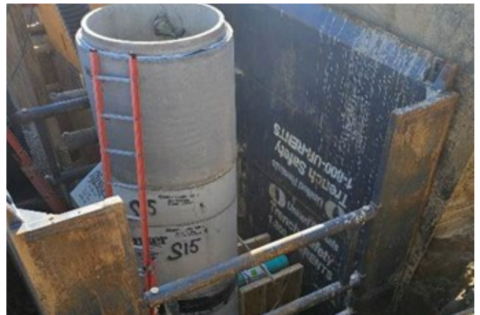
OUTSIDE DROP BEING INSTALLED AT PEABODY WEST
