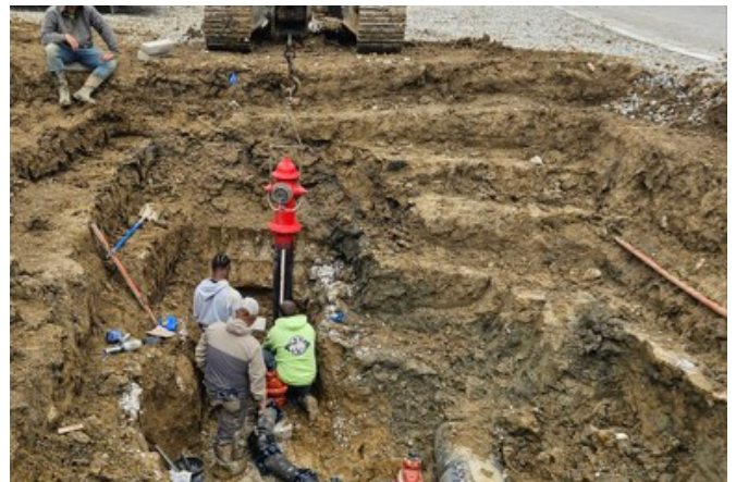
INSTALLING HYDRANT AT TACO BELL ON 267
