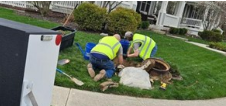
RAISING AND REPAIRING MAN- HOLES IN STONEGATE
