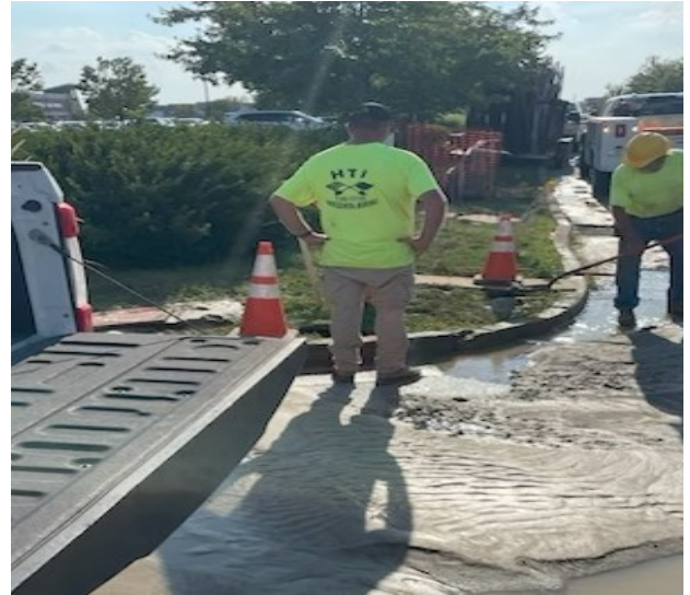
WATER MAIN REPAIR AT LOWES
